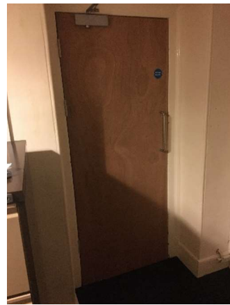
16. Typical basement door
