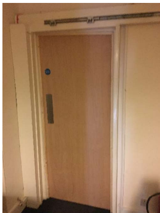
17. Typical basement door
