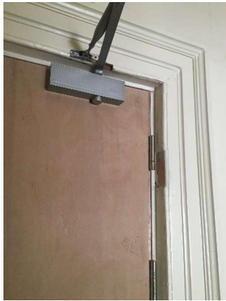
9. D1-2 closer/hinge detail
